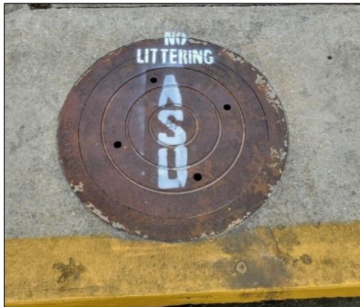
Figure 4. Example of ASU’s storm drain marking
