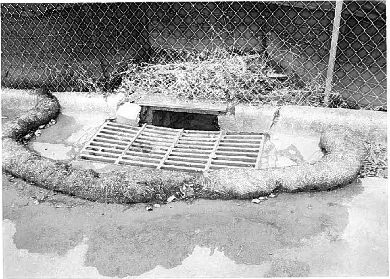
DORM - CLEAN DEBRIS
